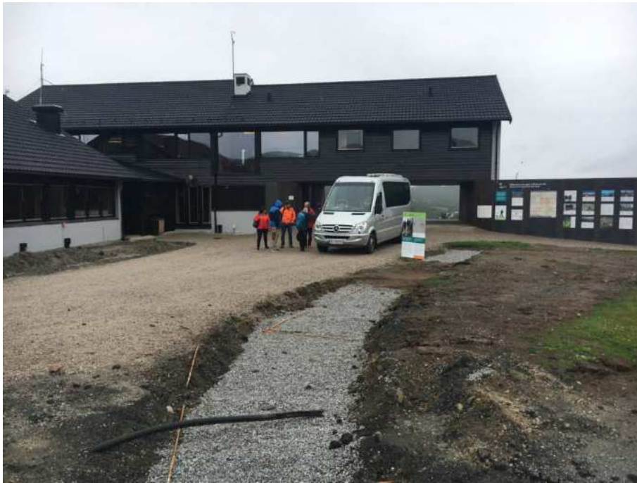
Photograph 16: The Wild Reindeer Centre (and National Park management hub) at Hjerkinn, repurposed former military buildings.
